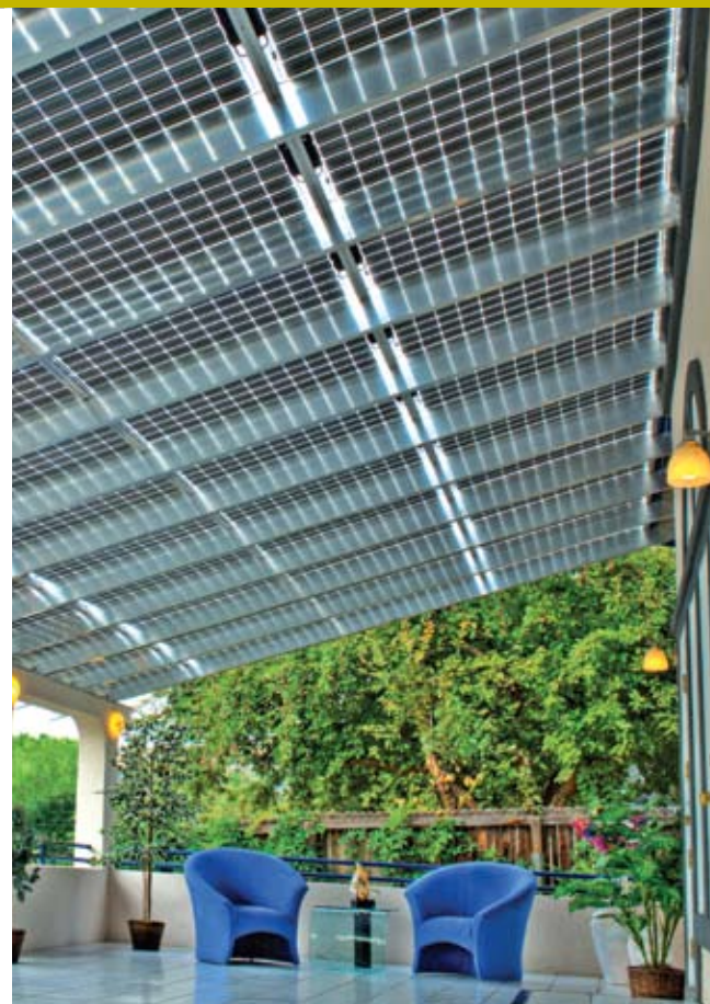
Patio Awning: 11.4kW Solar Living Design Lakewood, CO
