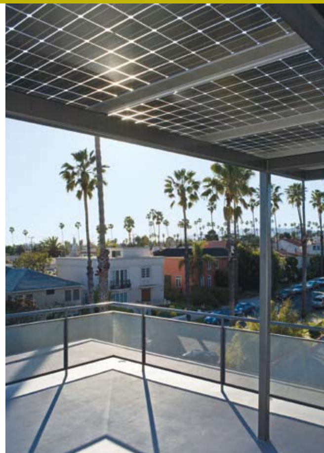
Rooftop Trellis: 1.95kW Golden Energy Inc. and Jesse Bornstein Architecture Santa Monica, CA
