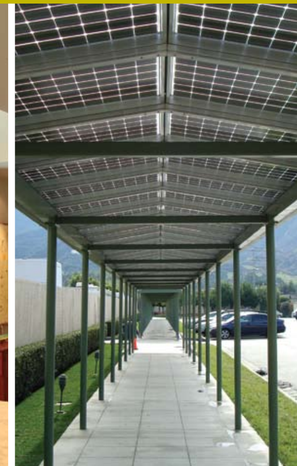
Breezeway: 44kW EI Solutions Burbank, CA
