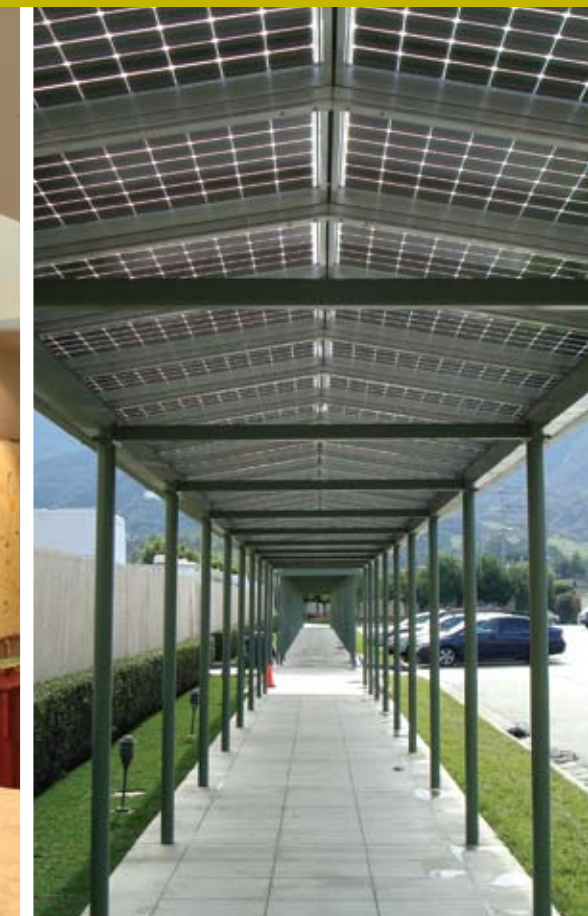
Breezeway: 44kW EI Solutions Burbank, CA
